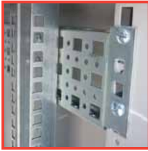
Horizontal Support Rail and 19" vertical Rail
